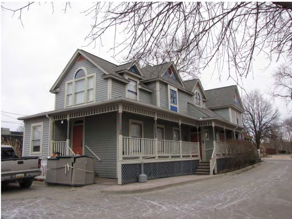
Main East 332_Looking Northwest
